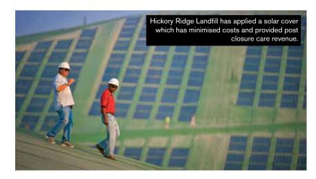
placed on top of the geomembrane product instead of the traditionally used soil and grass products.
